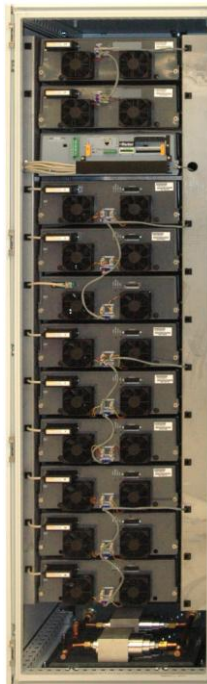
1 Megawatt inverter rack – Advanced Cooled
